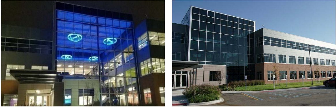
Figure 3 Trasparent and tinted states of thermochromic smart window in Masco Building facade (URL-3).
