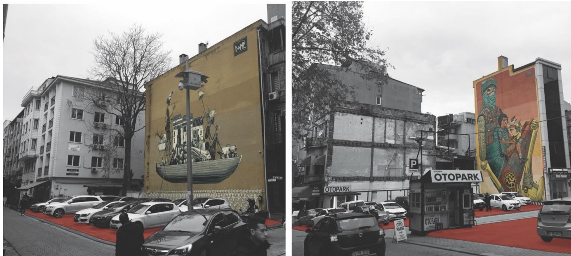
Figure 17 An observable match between the parking lots and the murals: such a coupling condition creates a characteristic setting.
