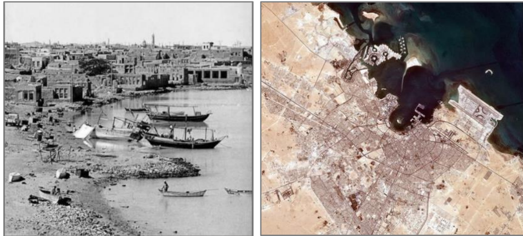
Figure 5 and 6: Doha's Evolution from a humble traditional settlement (1940s) to a metropolitan urbanity (2021) (Source: Courtesy of Ministry of Municipality).
