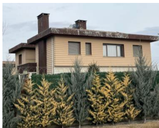
Figure 10 Northeast facade (Author 1, 2024)
