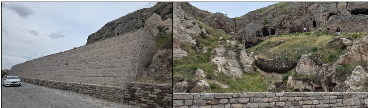
Figure 2 Photographs of rockfall mitigation measures, including stone walls and wire mesh applications, implemented in Sille to reduce rockfall hazard (From personal archive, June 1, 2025)
