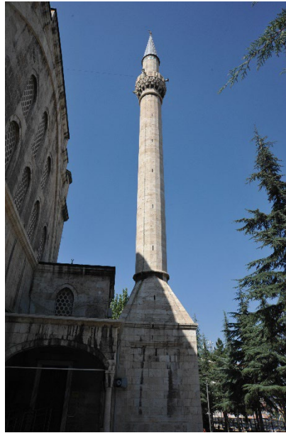
Figure 3 General view of Maltepe Mosque minaret
