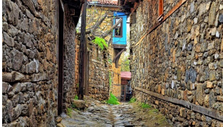
Figure 14 Timber ring beams in a masonry wall, Cumalıkızık, Bursa
