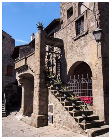
Figure 15 Outside staircase, (profferlo), Italy (Minor Sights, 2015)
