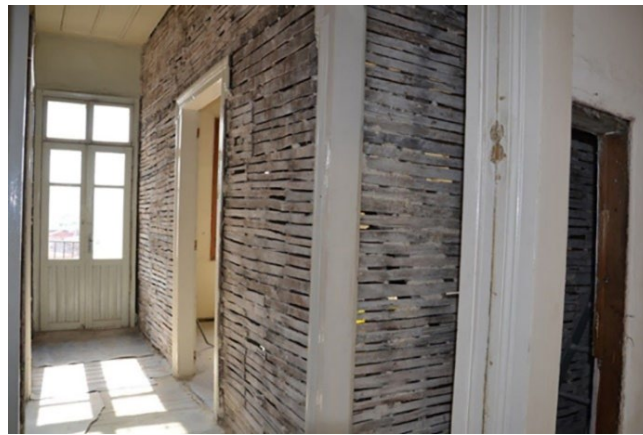
Figure 23 Lath and plaster ( bağdadi ) wall
