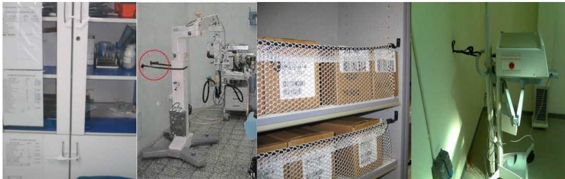
Figure 3 Precautions taken against non-structural risks in hospitals( parkzon, 2023 )
