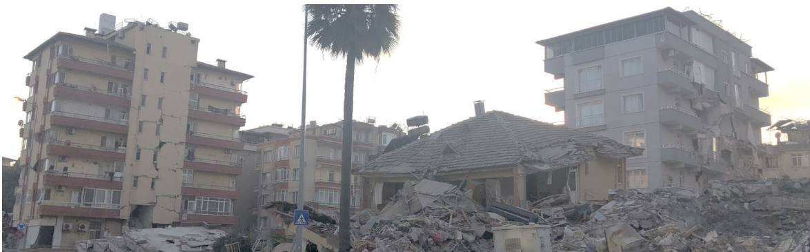
Figure 3 A view from the earthquake-hit area, Hatay, Türkiye.
