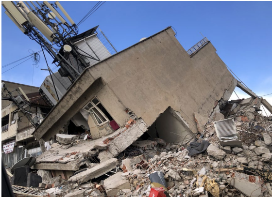
Figure 4a Damaged base station due to collapse of the building (photo from Kahramanmaraş).
