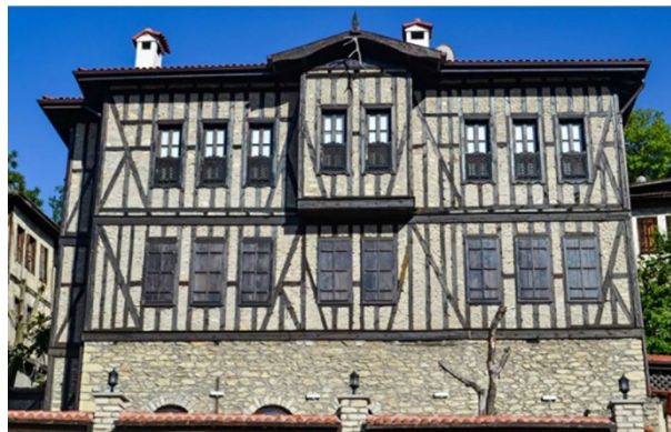
Figure 16 Diagonal bracings of an Ottoman House, Safranbolu, Karabük (BBC Travel, 2023)
