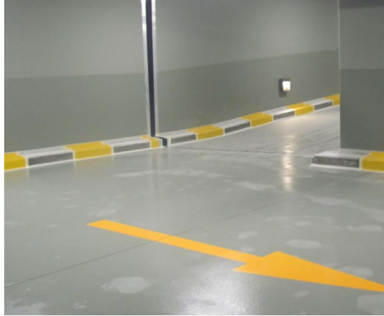
Figure 5 Example Wall and Floor Epoxy Application (Author Archive).
