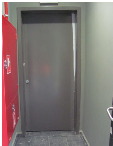
Figure 12 Fire Escape Door Installation Stage (Author Archive).
