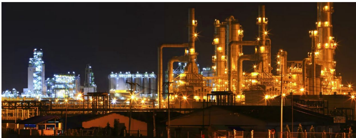
Figure 2 An Example of an Energy Facility ( https://proente.com )
