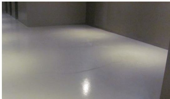
Figure 7 Sample Epoxy Application (Parting sand surface epoxy) (Author Archive).
