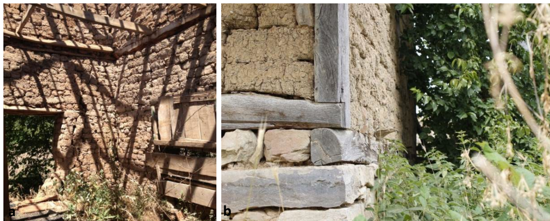
Figure 15 A Wooden beams and adobe blocks b Structure details in adobe system (photos: authors).
