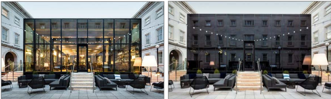
Figure 2 Transparent and tinted states of electrochromic smart window in Dirty Habit DC facade (URL-2).
