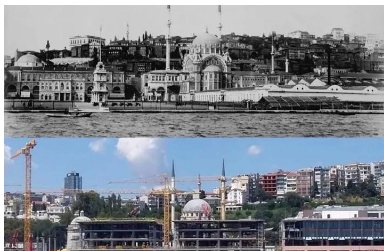
Figure 11 Impact of the project from the coastal area to the silhouette, the 1900s (top) and 2020 (bottom) (Url, 1).
