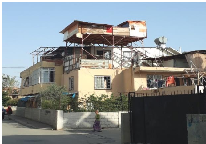
Figure 3 Housing constructions in the informal neighborhoods of Toroslar District
