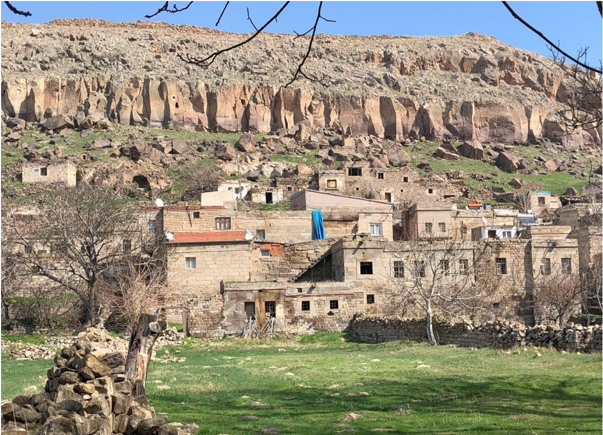
Figure 12 Basin settlement example from Mancusun (Gesi Valley)
