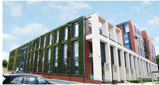
Photo 12 Living wall - educational building example with modular system application (URL -15)
