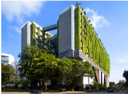
Photo 11 Green facade - Educational building example with wire mesh net system application (URL -14)
