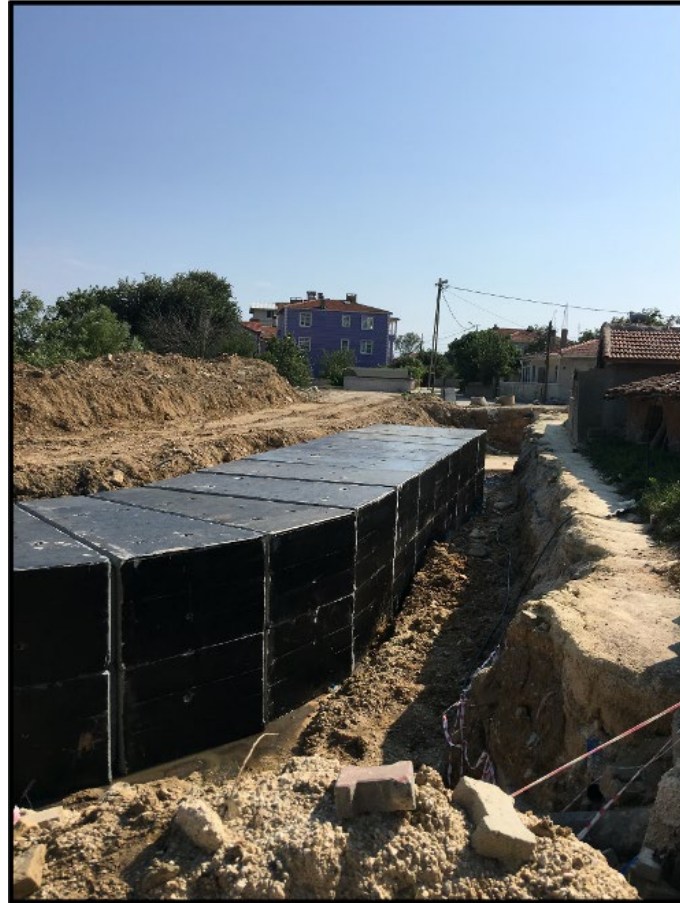
Figure 18 Rehabilitation Project of Akalan Stream (Author's own Archive, 2016)
