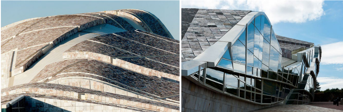
Figure 26a & Figure 26b City of Culture of Galicia, Spain (Eisenman Architects, n.d.)
