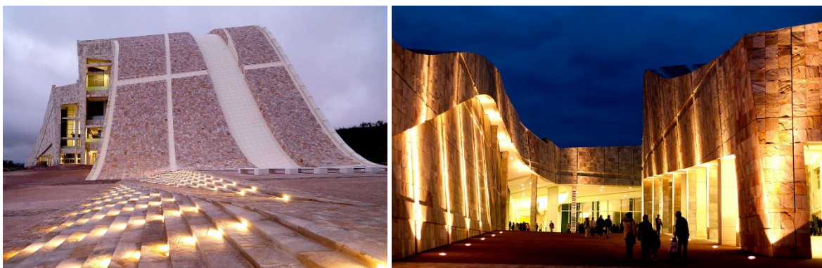
Figure 27a & Figure 27b City of Culture of Galicia, Spain (Eisenman Architects, n.d.)
