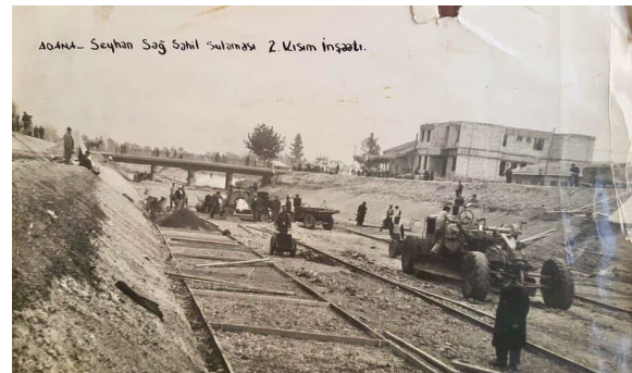
b. The process of concreting the irrigation canal, construction of Cemalpaşa Bridge and Bağlar Police Station, 1960s.
