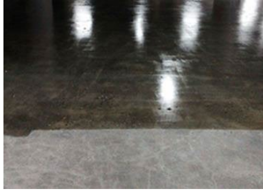
Figure 8 Sample Dust-Free Paint on Reinforced Concrete Flooring ( http://www.epoksizeminkaplamalari.com ).
